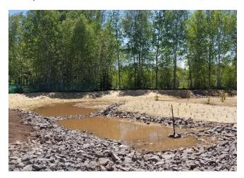
**Fun fact:** Forebays (above) can capture up to 50% of the sediment, trash and debris entering a green infrastructure site. Easy access for sediment removal reduces maintenance costs and preserves performance over time.
