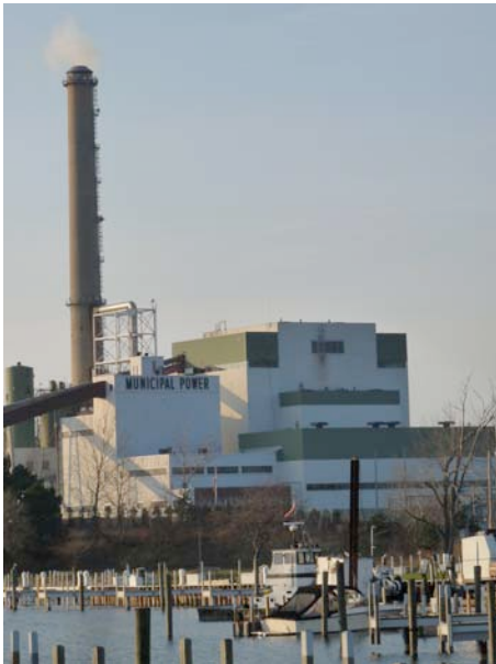
Figure 7a. Coal fired power plant in Grand Haven, MI. (E. Nordman)
