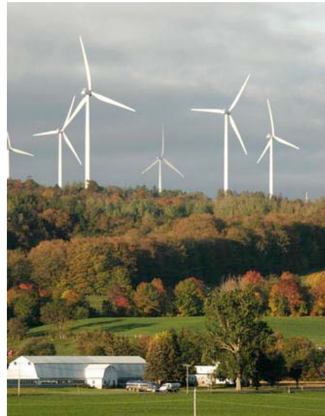
Figure 7b. Wind farm in New York with 83 turbines, each with a 260 foot tower and a capacity of 1.65 MW. (US Dept of Energy – NREL)
