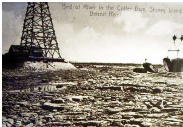
Figure 2. Detroit River Riverbed Dewatered Before Construction of the Livingstone Channel
