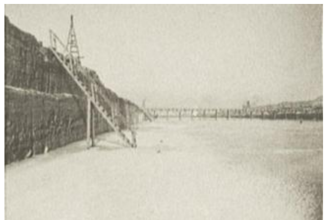
Figure 3. Detroit River Riverbed Dewatered After Blasting and Dredging of Shipping Channel
