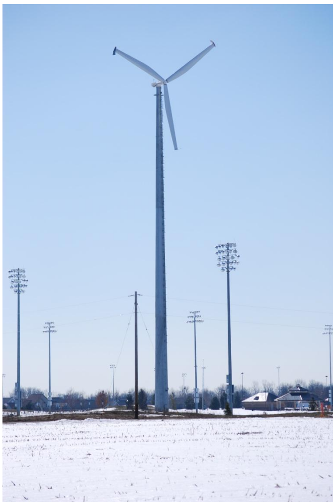
Figure 2. One of two 50 kW turbines in near Zeeland, Michigan. Each tower is 125 feet tall (Photo: J. VanderMolen).
