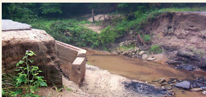
This rural road was completely washed out by an extreme storm on June 12, 2008. The Conservation Resource Alliance and Big Sable Watershed Restoration Committee are working to prevent this type of damage in the future.
