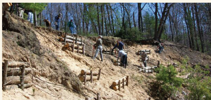
Volunteers work to terrace an eroding bank and install native plants on a Big Sable river bank. CRA and partners use these techniques to prevent erosion and protect fish habitat in the Big Sable watershed. Photos: Chris Pierce
