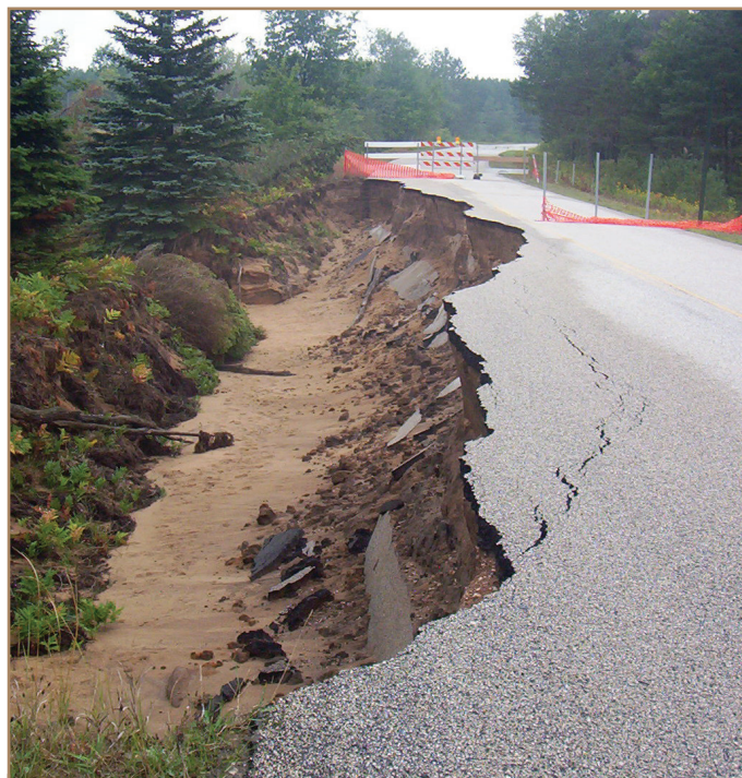
Road damage on Lake Michigan Drive near Ludington due to runoff from the June 12, 2008 storm that dumped 10 inches of rain in 12 hours. Photo: Chris Pierce
