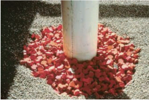
Figure 2: Scour protection, like this example from a bridge support column, is used to minimize erosion around the turbine foundation
