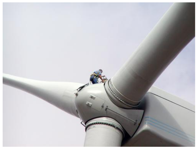
2b. Researcher entering the hub of a 1.5 MW wind turbine in Texas (GE Wind, TX, 2002). (US Dept of Energy – NREL)
