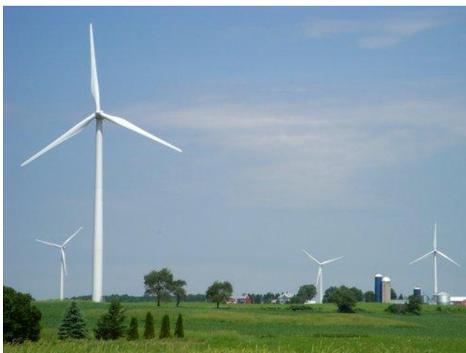
Figure 2a. Wind farm in Wisconsin with 86 turbines each at 1.5 MW capacity (Forward Wind Energy Center, 2009). (US Dept of Energy – NREL)
