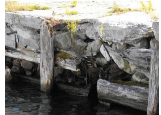
Damaged timber crib. Gene Clark
