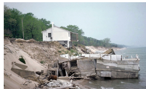
Coastal bluff failure. Erosion from waves, lakebed erosion and rainfall are the most common contributors to bluff failure or collapse. (Source: Michigan Sea Grant.)
