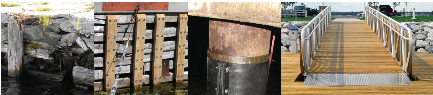
(L to R): Timber structure rot, timber crib repair and protective jacket for piling. Wood infrastructure is especially vulnerable to low water levels, which expose timber to oxygen that hastens deterioration. (Source: Gene Clark, Wisconsin Sea Grant.)
