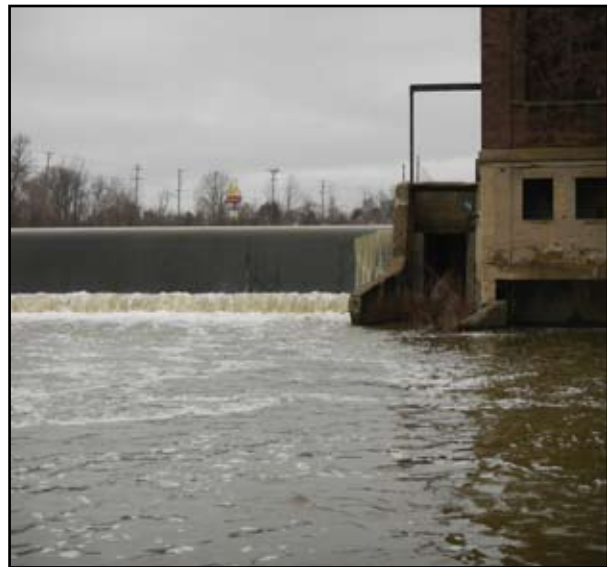
Peninsular Park Hyrdoelectric Structure
