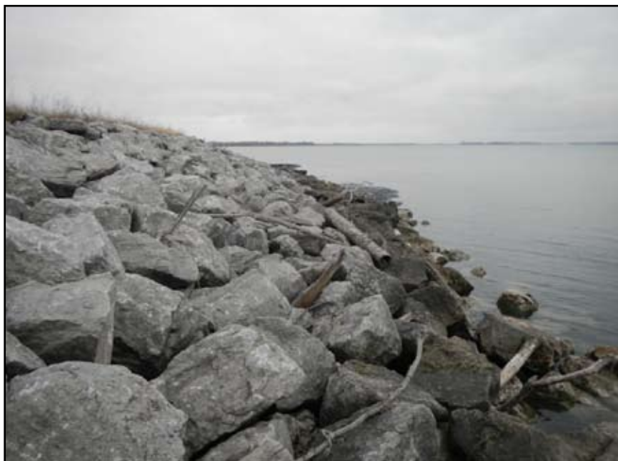
Limestone riprap dikes at Pointe Mouillee State Game Area.
