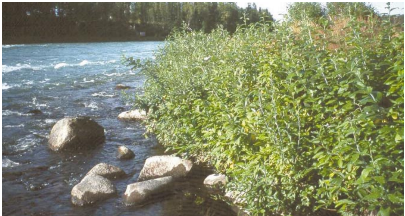
Figure 15 Large rocks placed in front of the live cribwalls provided additional fish cover.
