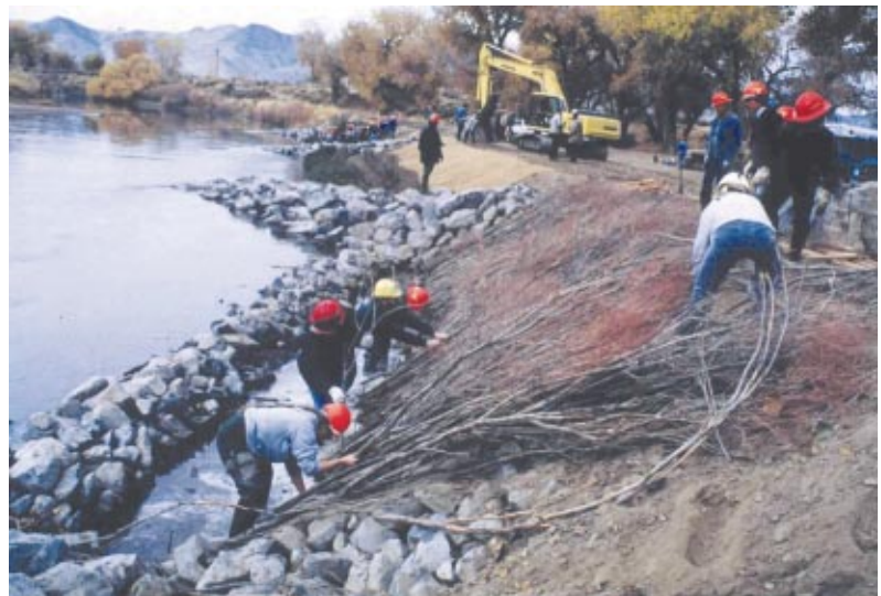
Figure 34 The willow brush trench between barb three and refusal. No erosion control blanket is used.
