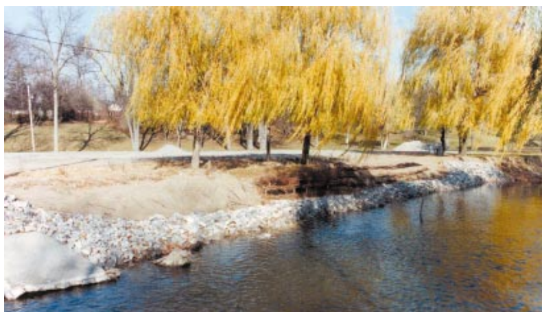
Figure 37 The workshop construction area where the three various techniques were used (from left to right: the brushmattress, vegetative geogrid, and live fascine).
