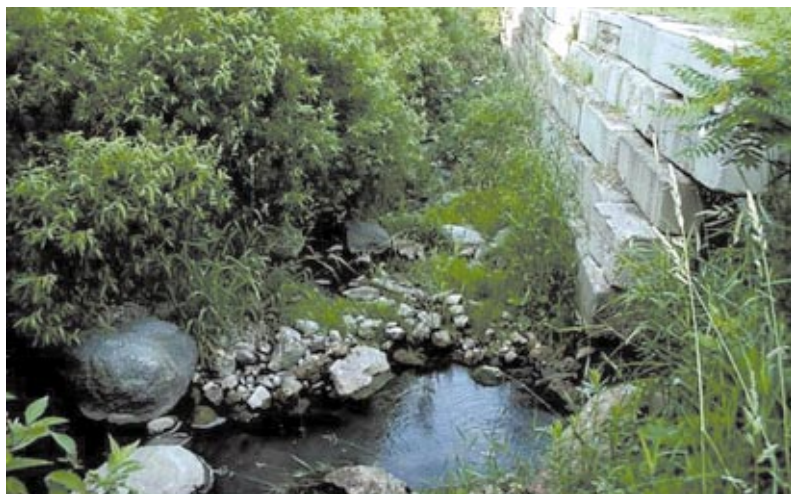
Figure 40 Deterioration of the concrete block wall, showing undermining and slumping of the structure on June 28, 2000.
