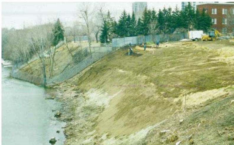
Figure 11 Placement of live fascines on contour with erosion control fabric along the Jacques Cartier Park.
