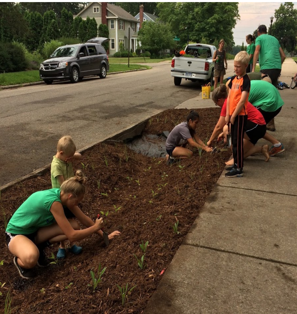
Curb Cut Rain Garden Installation with Green Team
