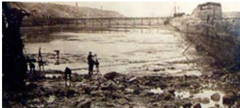
Construction of the Livingstone Channel in the Detroit River.
